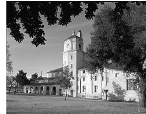
San Bernardino Valley College Auditorium Tower, circa 1933.
